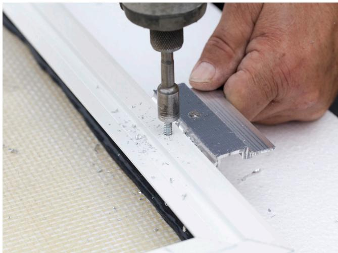
(installation direction is "up" and to the "right"). Holding the full clip firmly into the extrusion, drill a 5/32" hole through the panel extrusion into the full clip and continue through. Secure the clip with a #10 S.S. Pan Tek screw.
