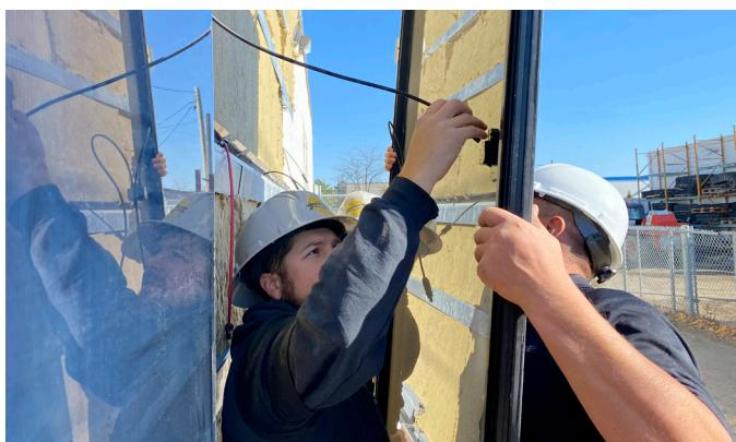
panel out to make any necessary electrical connections behind the panel. Check that the panel is level, recheck panel to the laser line previously marked on the wall.
