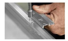
3 To speed up installation, attachment clips can be installed to the panel perimeter to align with the sub-framing locations.
