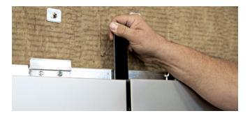
**9 Vertical** infill strips are measured and installed once a row of panels are installed.
