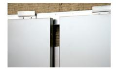
7 **Repeat steps 3-5.** The next panel is placed onto the J-trim and slid over to connect with the previous panel installed.
