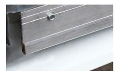
J-trim is mounted to the sub-framing at the base of the wall over top of the flashing.
