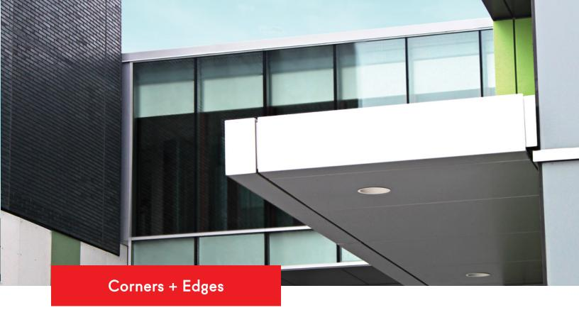
It's recommended that installation begins at a corner or window jamb. Corner and window jamb panels are custom cut and constructed based on approved shop drawings.
