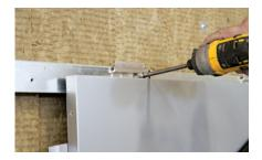
6 The full clip is attached to the sub-framing using a self-taping hex screw with an extended hex head driver.
