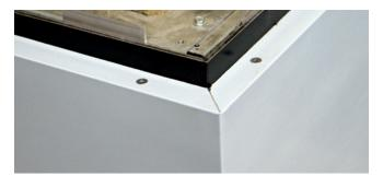
Infill strips can be routered from the back and bent to create a clean corner.
