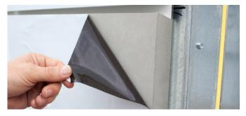
Once the installation is complete, the Alumitex<sup>®</sup> protective dust-cover can be removed from the panels.
